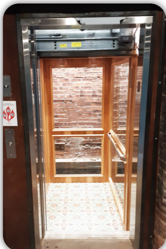
LULA with Flat panels in Hickory Clear coat prepped for glass (glass by others).
