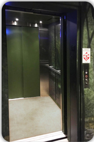
LULA with custom laminate applied panels and field painted doors.
